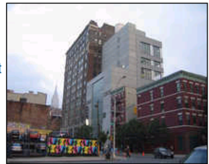
The ARTS Building at 450 West 37th Street
